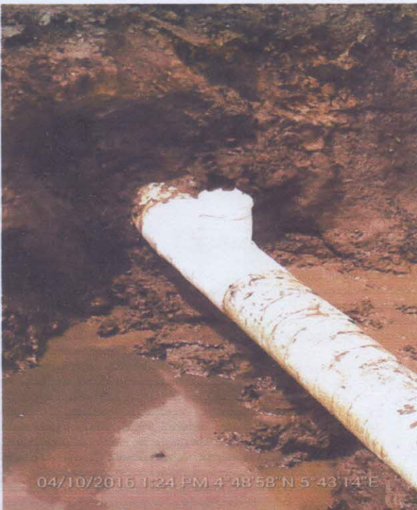
Fig 4: Repaired point wrapped
